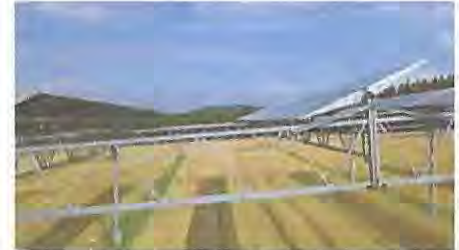
Pilot plant at Heggelbach Farm in Germany, where different crops are grown under PV modules
